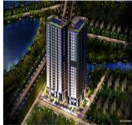
Hateco Address: Hoang Mai, Ha Noi No. of Elevator : 10 units Max Speed : 120 mpm Max Load : 1000 Kg Max Stop : 28 Stops
