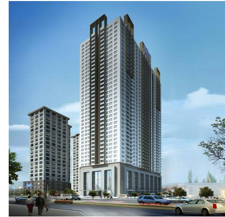
CT4 Vimenco Address: Trung Hoa, Cau Giay, Ha Noi No. of Elevator : 12 units Max Speed : 180 mpm Max Load : 1150Kg Max Stop : 43 Stops
