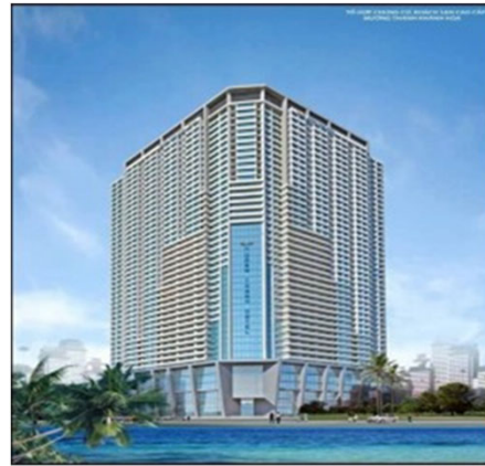
Muong Thanh Khanh Hoa Address: Nha Trang, Vietnam No. of Elevator : 14 units Max Speed : 180mpm Max load : 1600 kg Max stop : 48 stops
