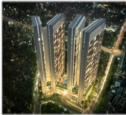
Dolphin Plaza Address: Nam Tu Liem, Ha Noi, No. of Elevator : 6 units Max Speed : 180 mpm Max Load : 1350 Kg Max Stop : 28 Stops
