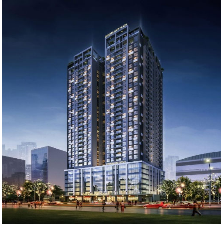
DREAMLAND BONANZA Address: Duy Tan, Cau Giay, Ha Noi No. of Elevator : 12 units Max Speed : 150 mpm Max Load : 1000Kg Max Stop : 36 Stops
