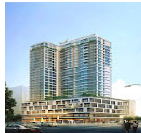
Muong Thanh Phu Tho Address: Phu Tho, Vietnam No. of Elevator : 9 units Max Speed : Max load : Max stop :
