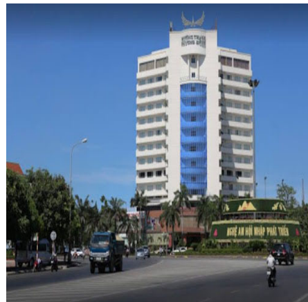
Muong Thanh Cua Dong Address: Nghe An, Vietnam No. of Elevator : 8 units Max Speed : 150mpm Max load : 1350 kg Max stop : 28 stops
