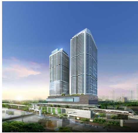
D32 CAU GIAY COMPLEX Address: Cau Giay, Ha Noi, Vietnam No. of Elevator : 6 units Max Speed : 2.0 m/s Max Load : 1600 Kg Max stop : 29 stops
