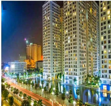
HH2 Linh Dam Address: Hoang Mai, Hanoi No. of Elevator : 18 units Max Speed : 180 mpm Max Load : 1350 Kg Max Stop : 42 Stops
