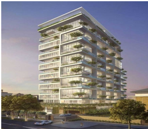
Serenity Address: Dist. 1, HCMC, Viet Nam No. of Elevator : 7 units Max Speed : 120 mpm Max Load : 1150 Kg Max Stop : 19 Stops
