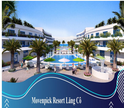
MOVENPICK LANG CO RESORT Address: Da Nang, Viet nam No. of Elevator : 8 units Max Speed : 60 mpm Max Load : 1000 Kg Max Stop : 4 Stops
