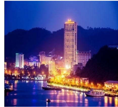
Muong Thanh Son Tra Address: Da Nang, Viet nam No. of Elevator : 24 units Max Speed : 180mpm Max load : 1350 kg Max stop : 42 stops
