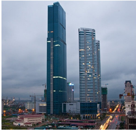
Keangnam Landmark Tower Address: Nam Tu Liem, Ha Noi, Vietnam No. of Elevator : 20 units Max Speed :210 mpm Max load : 1350 Kg Max stop : 72 Stops
