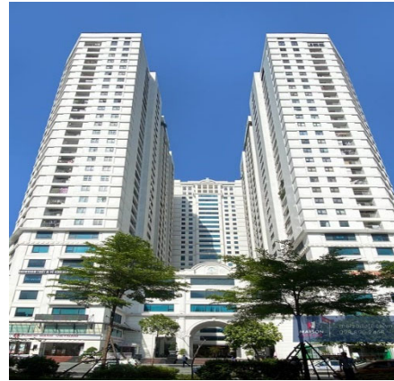
219 Trung Kinh Address: Cau Giay, Ha Noi No. of Elevator : 17 units Max Speed : 180 mpm Max load : 1350 Kg Max stop : 34 Stops
