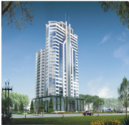
Viwa Seen Trung Van Address: Trung Van, Ha Noi No. of Elevator : 14 units Max Speed : 2.0 m/s Max Load : 1600 Kg Max stop : 28 stops
