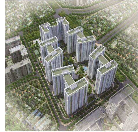
ECOHOME 3 Address: Tu Liem, Ha Noi, Vietnam No. of Elevator : 28 units Max Speed : 2.5 m/s Max Load : 1350 Kg Max stop : 37 stops
