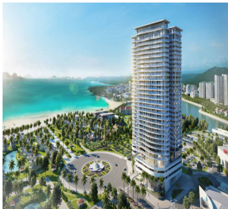
CITADINES MARINA HA LONG Address: Ha Long, Quang Ninh No. of Elevator : 14 units Max Speed : 180 mpm Max Load : 1600 Kg Max Stop : 34 Stops
